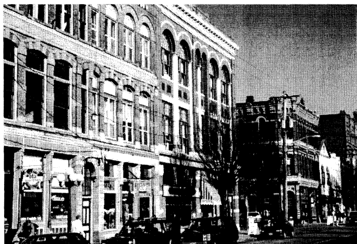
Liberty's offices on Water Street in downtown Port Townsend
